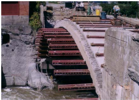
Forming for Downstream Sidewall
