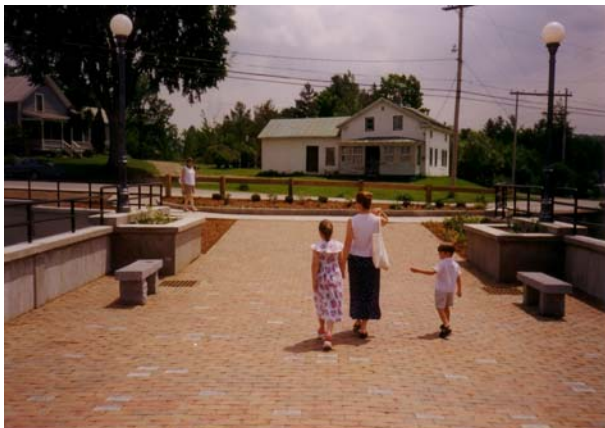
Brick Surface and Concrete Planters
