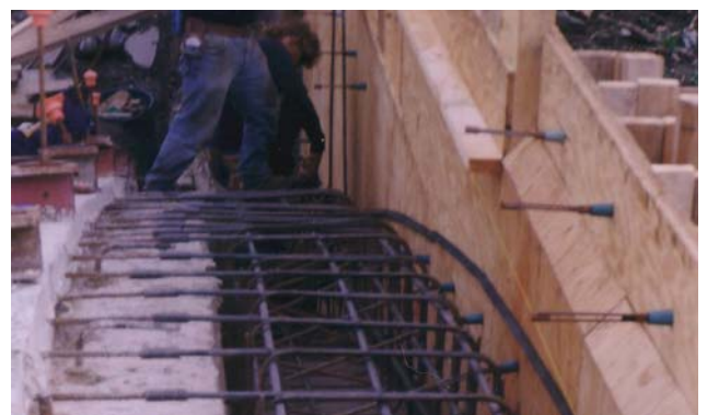
Reinforcing for Arch Below the Downstream Sidewall
