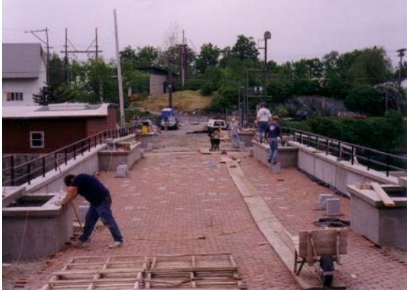
Setting Brick Pavers
